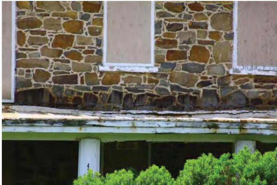
Deterioration Of Front Porch Roof Framing
