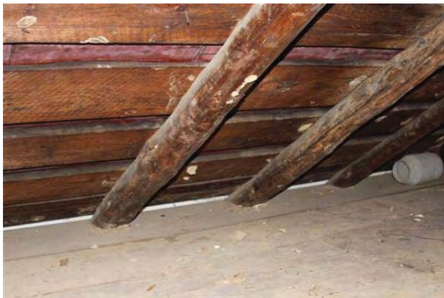
Rafter Connection At Attic Floor
