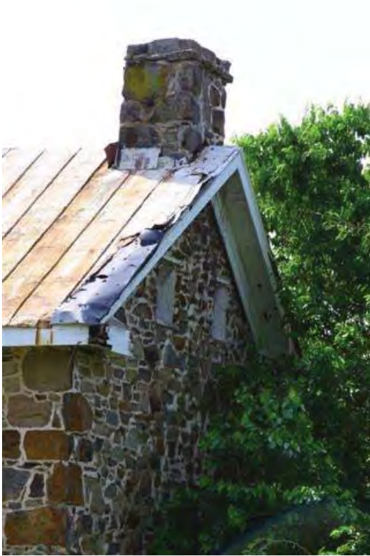
Chimney Displacement On Right Side Of House
