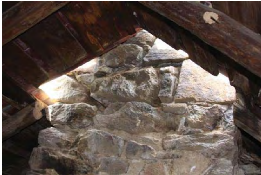
Gap Between Roof And Chimney – Right Side
