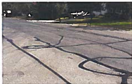
Roadway after cracks are sealed, but before slurry application.
