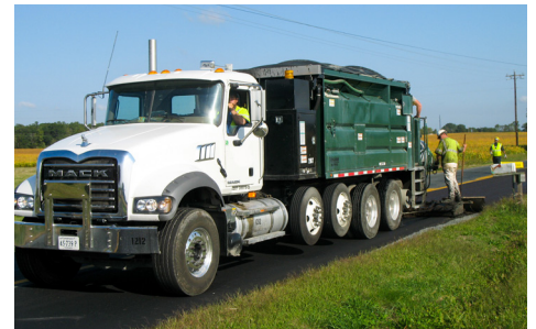
Typical truck used in slurry seal operations.
