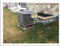
**Solution:** In order to eliminate the possibility of damage, we recommend removing the turf on all sides of the AC/heat pump unit and install river rock around the unit extending it out to at least 6 inches on all sides. Not only is this aesthetically pleasing to prolong the unit, but it will also alleviate debris, such as dirt and mulch, to be sucked into the unit.
