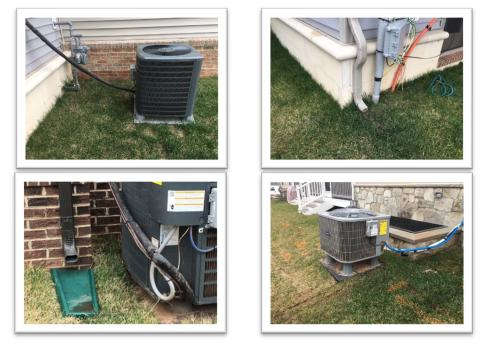
**Solution:** To eliminate the possibility of damage, we recommend removing the turf on all sides of the AC/heat pump unit and installing river rock around the unit extending it out to at least 6 inches on all sides. Not only is this aesthetically pleasing to prolong the unit, but it will also alleviate debris, such as dirt and mulch, to be sucked into the unit.
